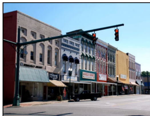
Commercial row on north side of the square
